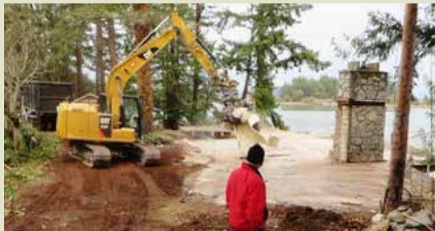
Above: A Trust volunteer watching as the house is removed.
