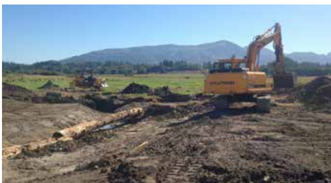
The same spot one year earlier, as crews work to re-meander the creek.
